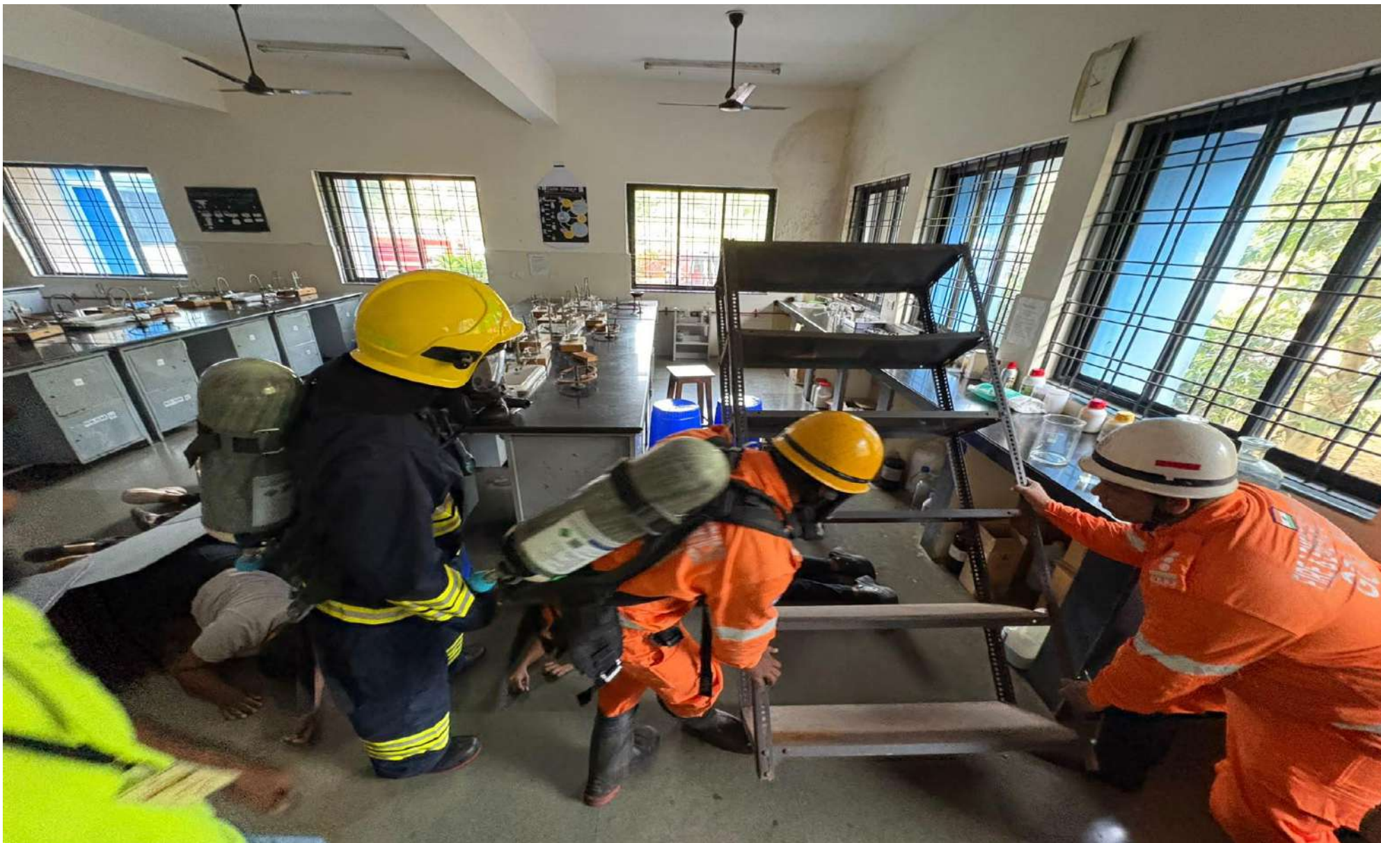
Ponda Fire Station: Incident: Partial roof collapse at the pharmacy college, Farmagudi.
